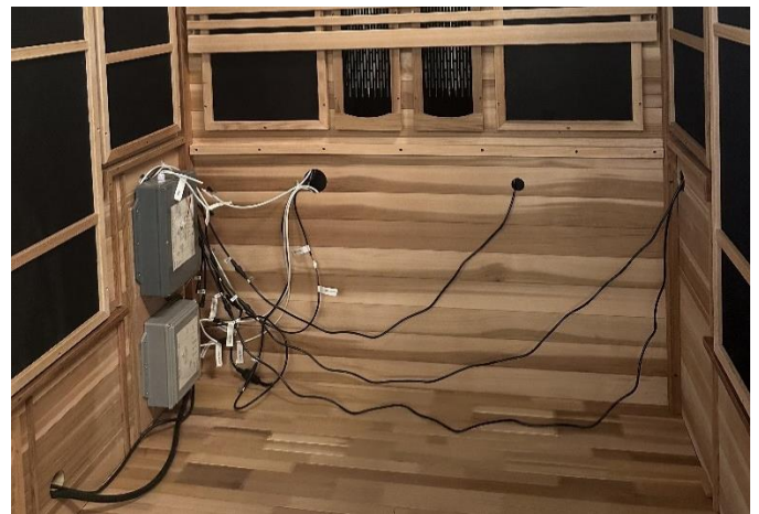
Figure 6 Please note that the junction boxes are on the REAR WALL PANEL for GDI-8523-01 and LEFT SIDE WALL PANEL for GDI- 8526-01.
